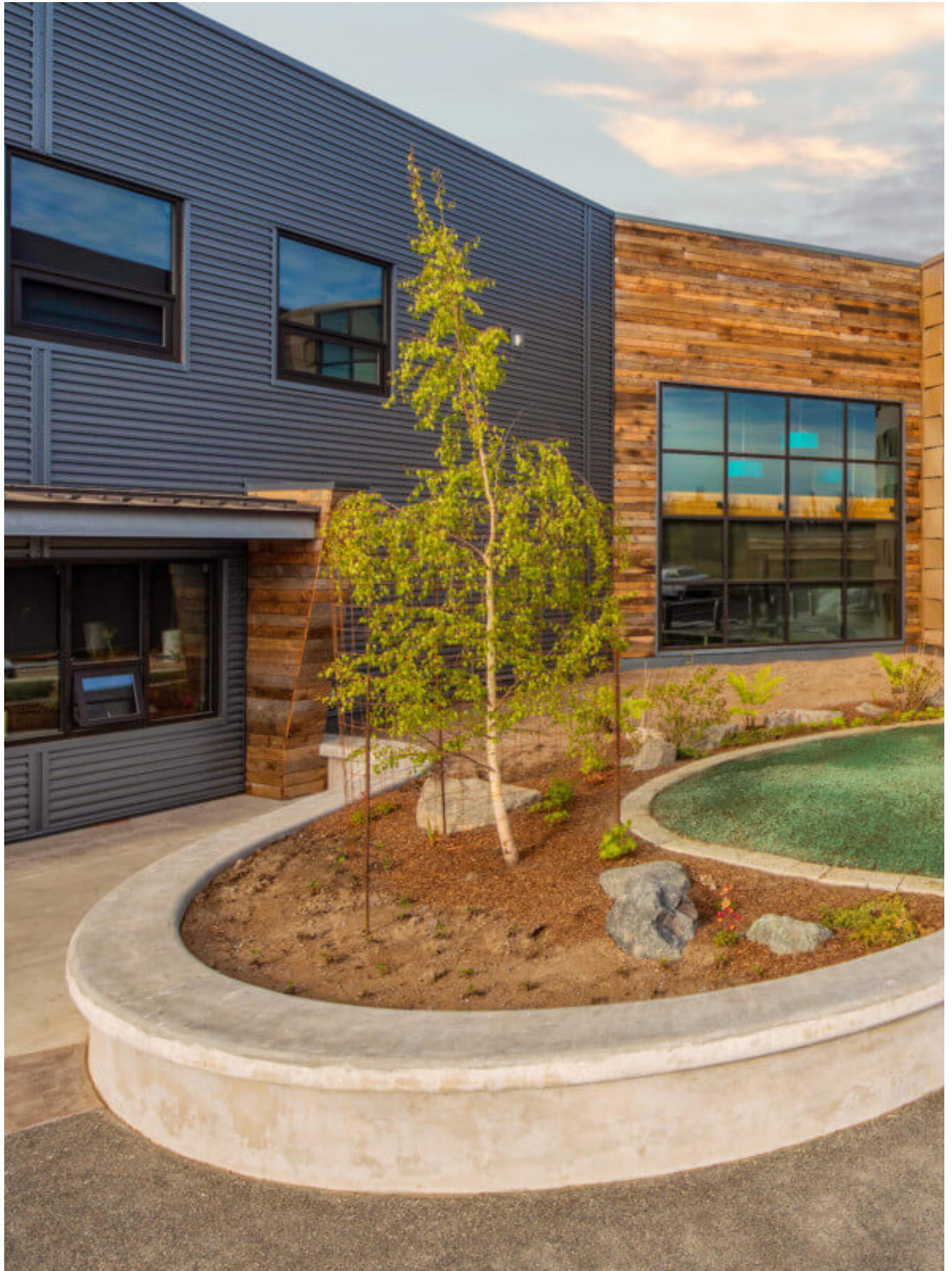
The combination of metal paneling and wood can be seen in contrast on the facade. (Wayde Carroll)
